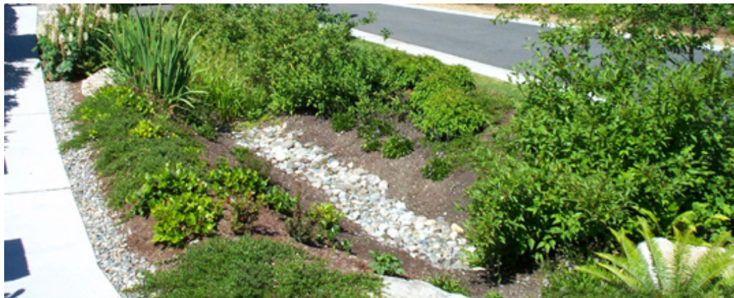
Consider using vegetated swales and other stormwater best management practices
