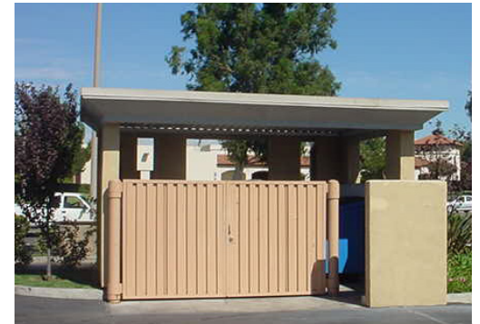
Pedestrian entrances to trash enclosures are recommended
