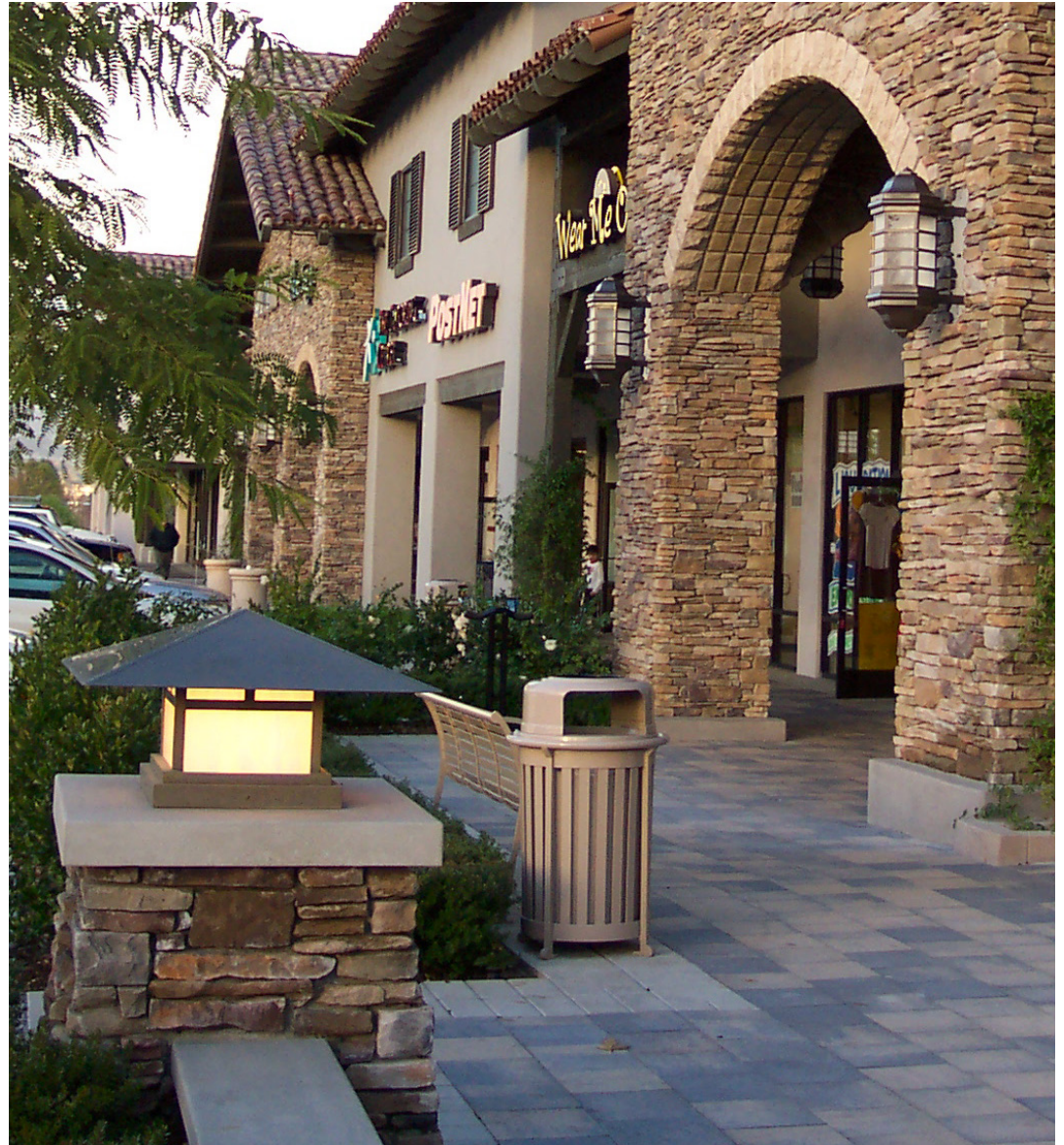
A variety of lighting options provides visibility and enhances architectural details
