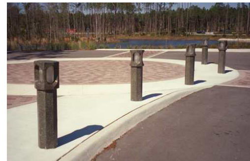
Bollards with light elements can be used to provide subtle lighting
