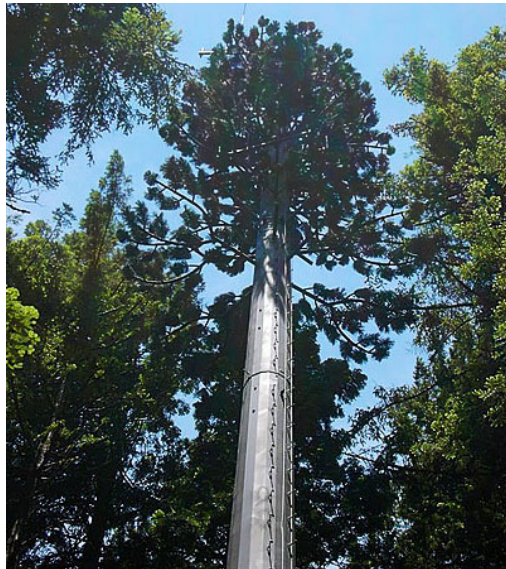
Antennas designed to match existing trees can create an attractive alternative to traditional antenna sites
