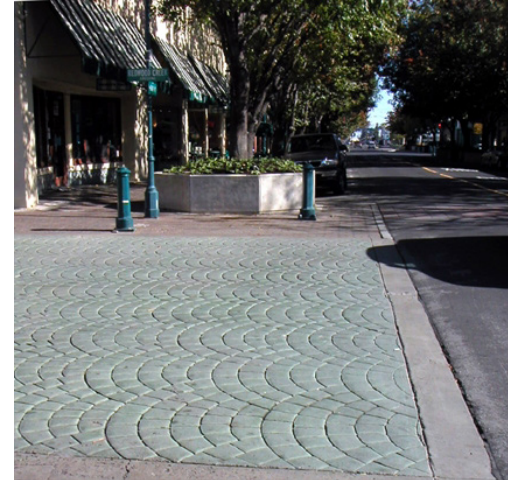
Accent paving enhances the crosswalk and alerts drivers to the likely presence of pedestrians
