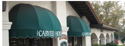
Awnings should be well maintained
