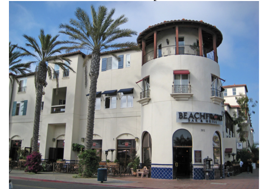
Example of a mixed use development
