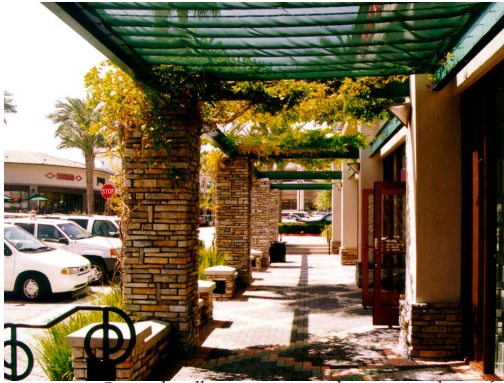
Covered walkways can provide a protected area for pedestrians
