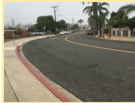
Existing conditions at Libby Elementary School
