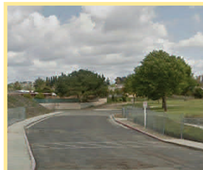
Sidewalk Gap at Parking Lot Entrance
