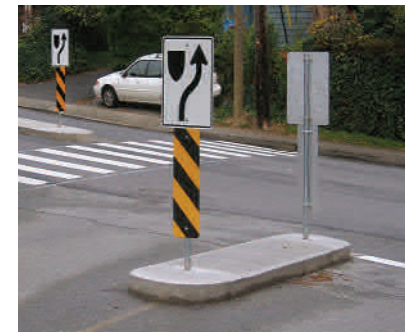
Traffic Calming Median
