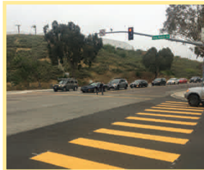
Existing crosswalk at Martin Luther King Middle School
