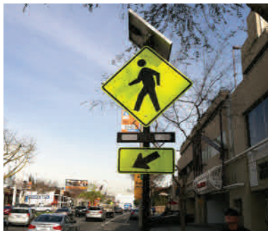
Rectangular Rapid Flashing Beacons (RRFB)
