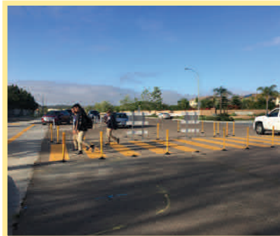
Existing crosswalk at Mission Vista High School
