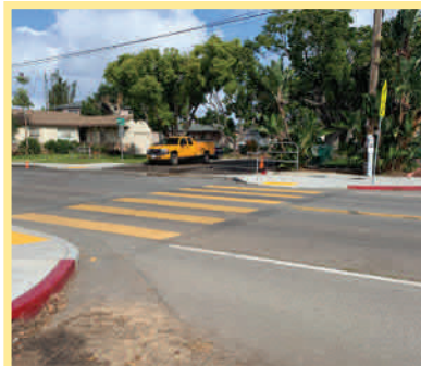
Existing crosswalk at South Oceanside Elementary School
