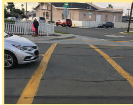
Existing crosswalk at Laurel Elementary School
